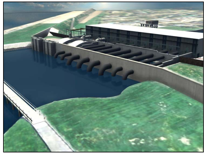
Pump station with Fronting Protection in place.
