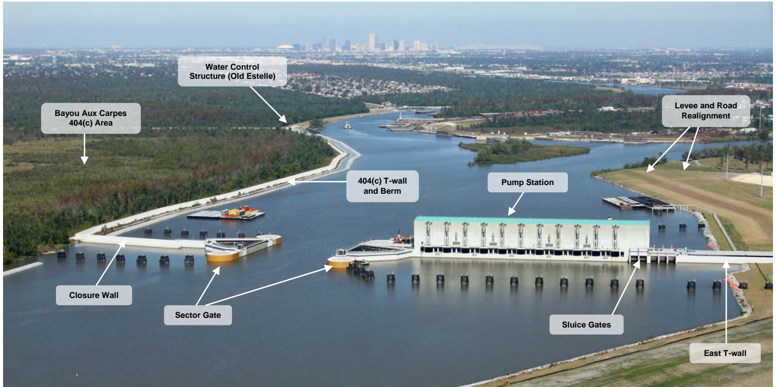
Image of the GIWW-West Closure Complex
