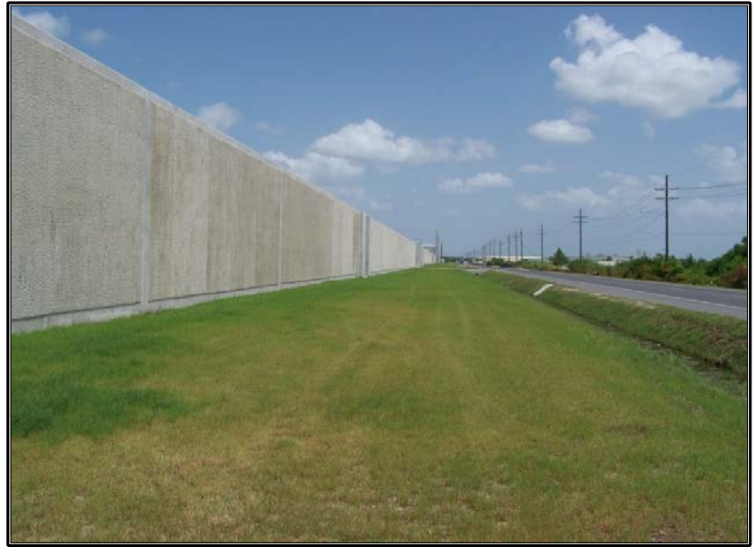
View of the Harvey Canal Floodwall along Peters Road.
